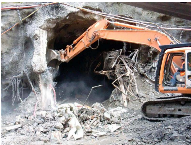
A digger removes the portal seal. Photo: NZPA.
